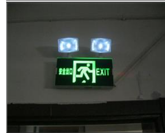
Photo of fire safety equipment Test of the emergency lighting and exit sign.JPG
